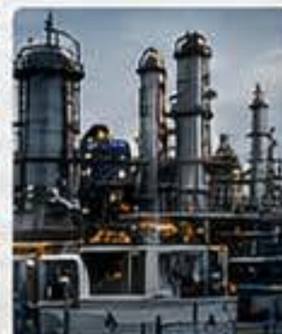
ENERGY & POWER SYSTEMS
