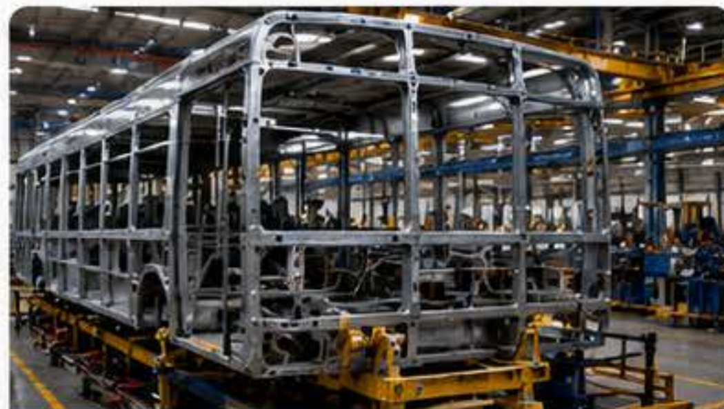
BUS FRAME FABRICATION
